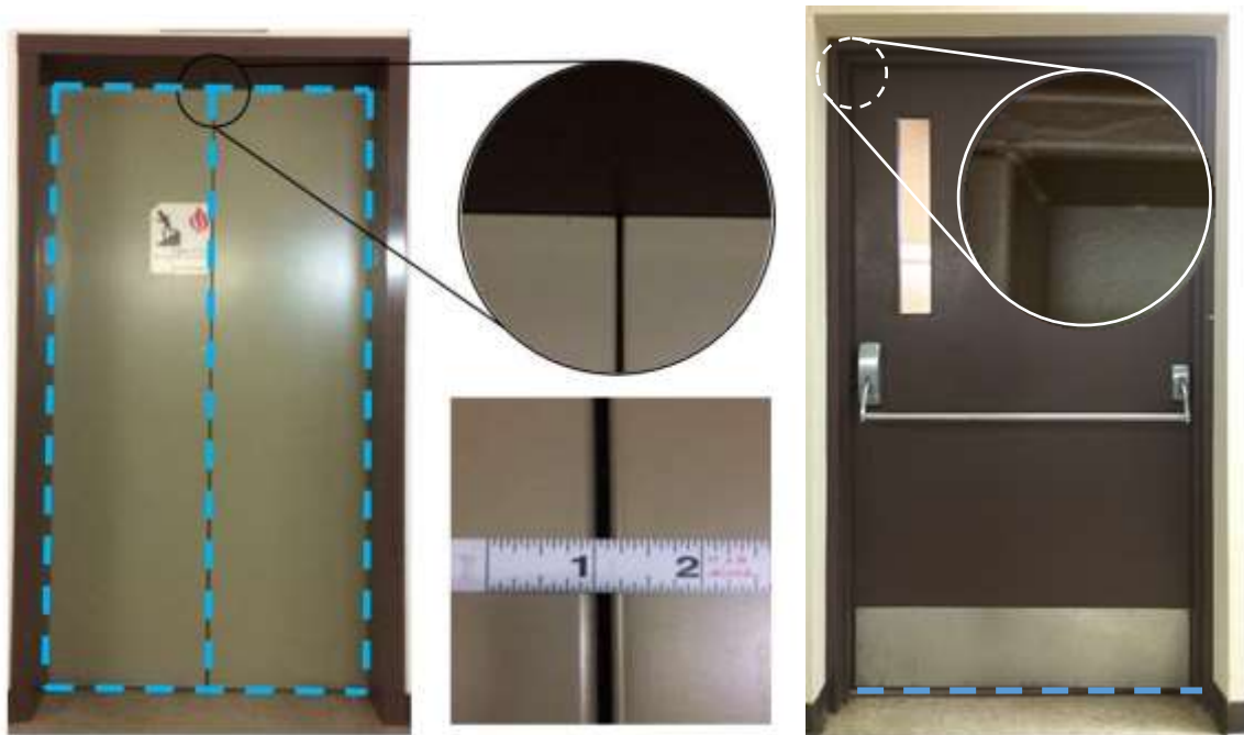
Figure 5 Leakage area locations of a typical passage elevator door (left) and stair door (right) in office buildings
