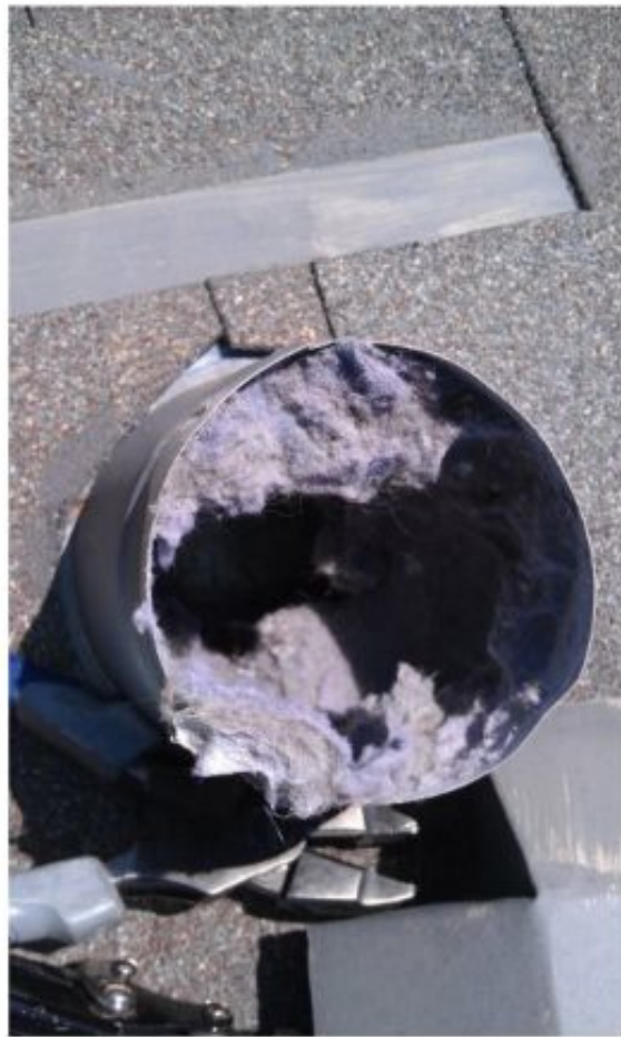
Examples of vent caps that duct cleaners wrongly disassemble to gain access.
