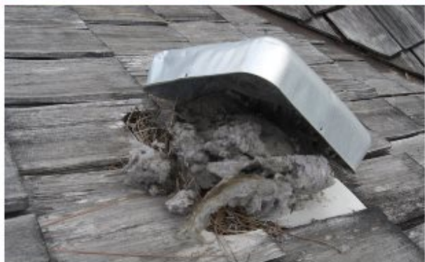
Examples of vent caps that duct cleaners wrongly disassemble to gain access.
