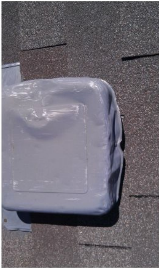
Examples of vent caps that duct cleaners wrongly disassemble to gain access.
