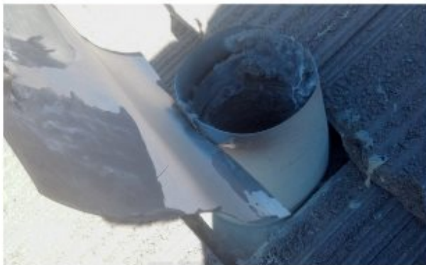
Examples of vent caps that duct cleaners wrongly disassemble to gain access.
