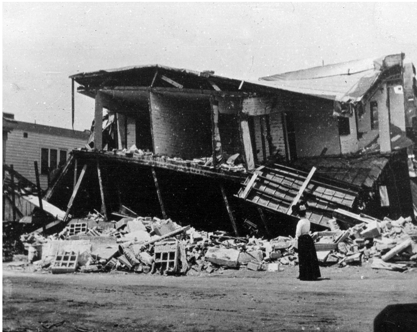
View of damage to a frame house in San Francisco as a result of the earthquake of 1906.
