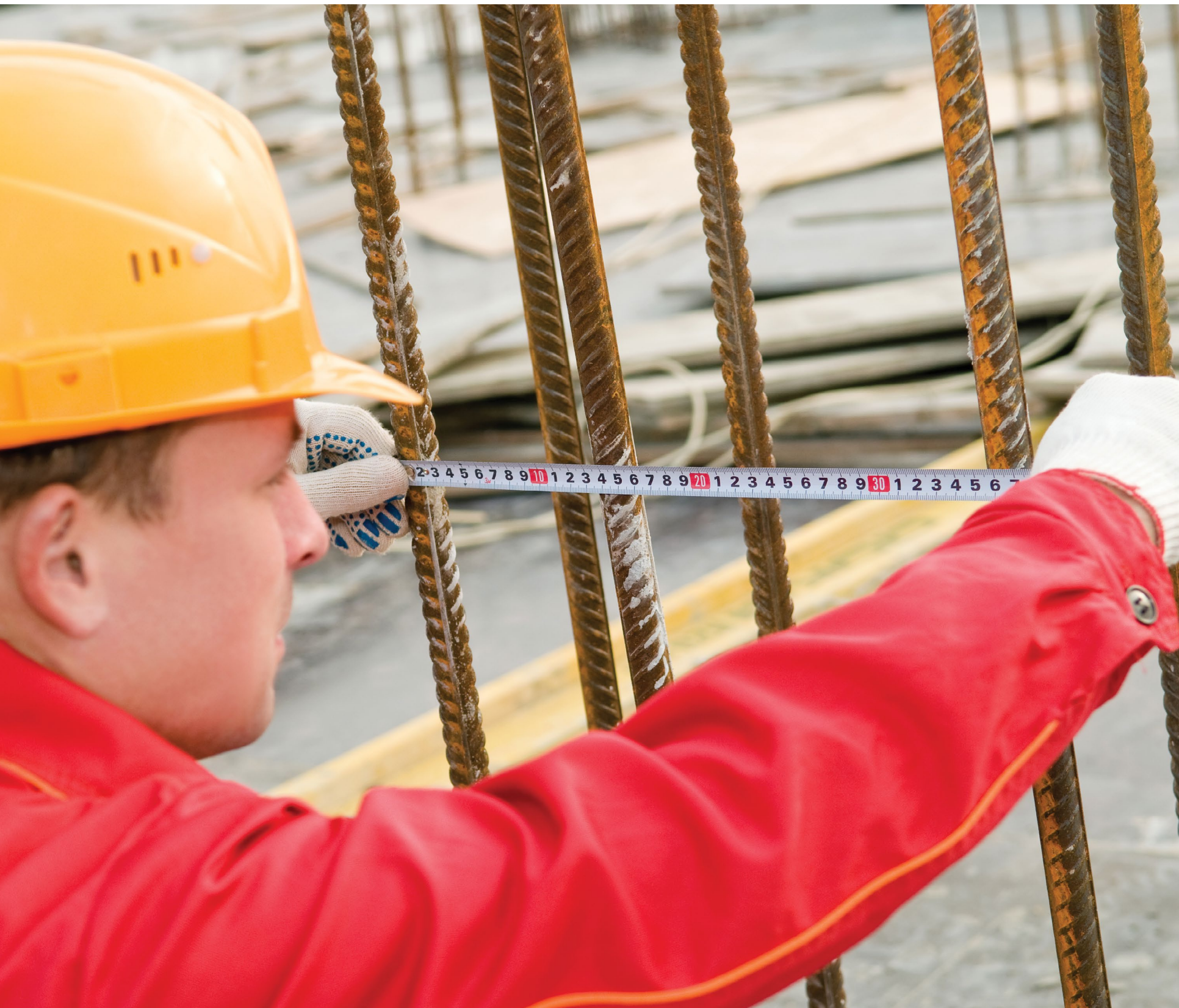
Worker measures the distance between reinforcement bars at a construction site.
