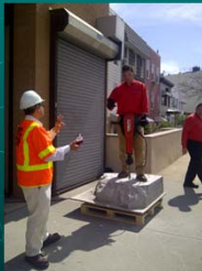
Electric pavement breaker
