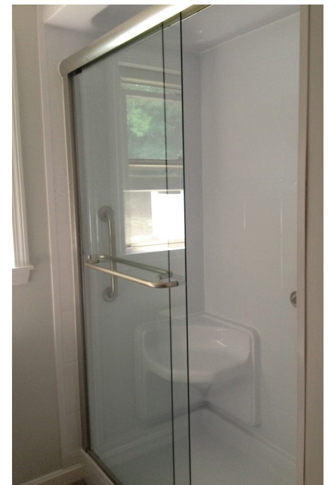
New walk-in shower, adjustable shower head, shower seat, and horizontal and vertical grab bars.
