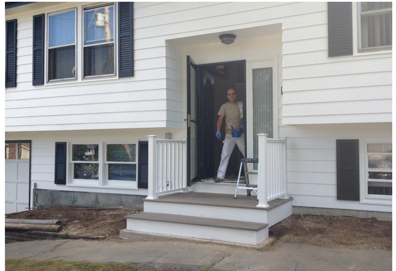
New front stairs and landing with proper rise and run.
