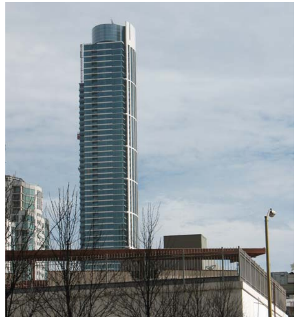
San Francisco's One Rincon Hill complex comprises two high-rise condominium structures designed using performance-based procedures.
