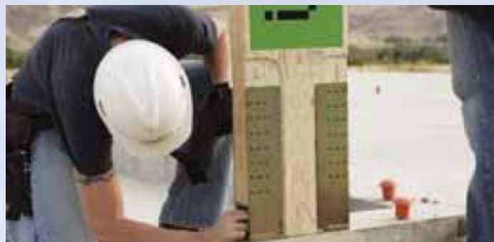
Shear Brace Portal Frame
