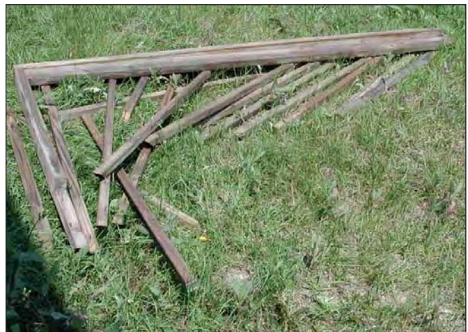
The aftermath of an incident in which a young man died after falling through a guardrail that was nailed only to joists on the end of the deck.
