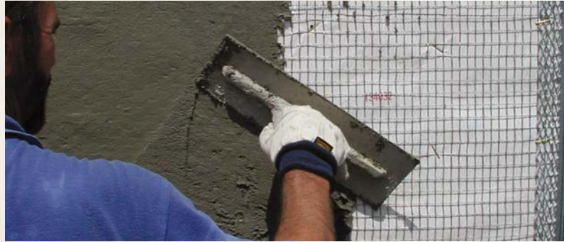
Self-furring PermaLath enables stucco keying.
