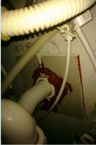
This is an example of where the fire-caulking material has not been properly tooled as the material has not been evenly distributed around the opening.
