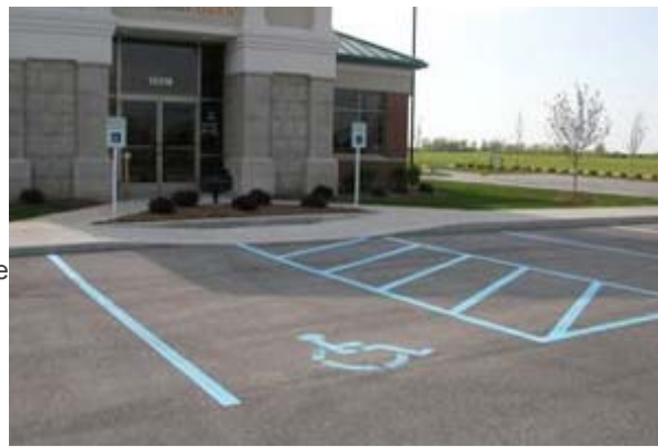
Figure 5: Curb solution with depressed sidewalk
