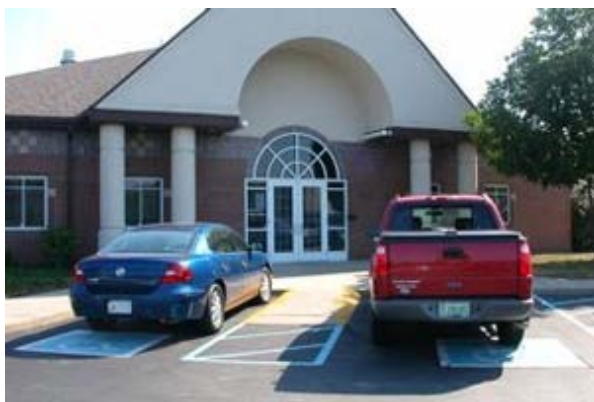
Figure 2: A built-up curb cut ramp overlapping access aisles.
