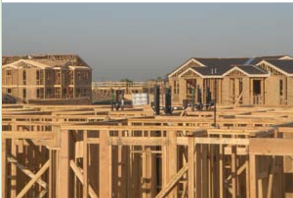
The venting system (center) advances skyward along with the construction.
