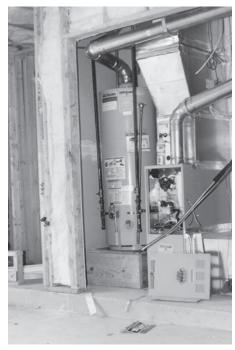
The illustration of an elevated water heater in a garage indicates proper planning during construction for adequate servicing and replacement at a later date. Doors may be added at a later stage of construction and will not be considered as permanent construction if the appliance needs to be replaced later.
