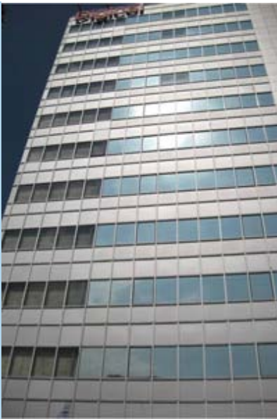
Digicel headquarters in Port-au-Prince, Haiti after the earthquake. The building suffered some very minor damage, but is essentially intact. Photo by Dr. Reginald Desroches.
