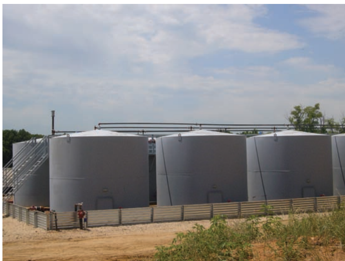
FIGURE 1-13 The design of these petroleum storage tanks was required by the fire code official to comply with one of the atmospheric storage tank design and construction standards developed by the American Petroleum Institute
