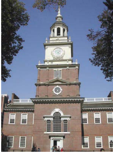
FIGURE 1-12 Historic buildings must comply with a fire protection plan approved by the fire code official
