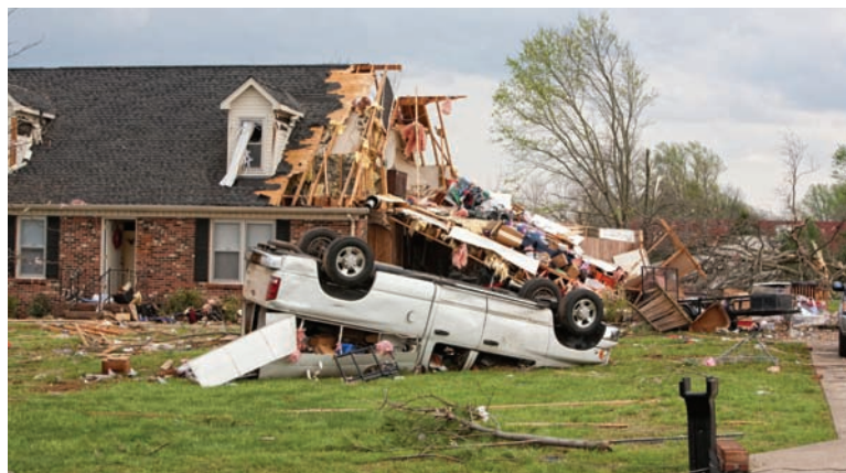
FIGURE 4-10 Tornado damage (Courtesy of iStock)
