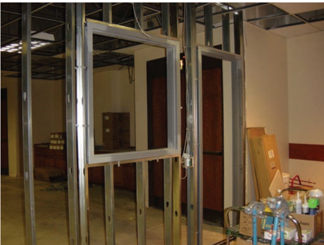
FIGURE 2-9 Cold-formed steel light-frame construction framing
