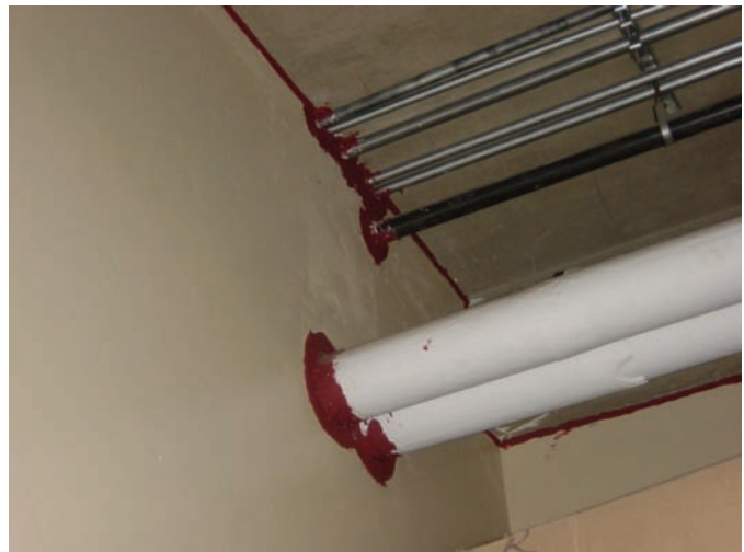
FIGURE 2-10 Through-penetration fire-stop system
