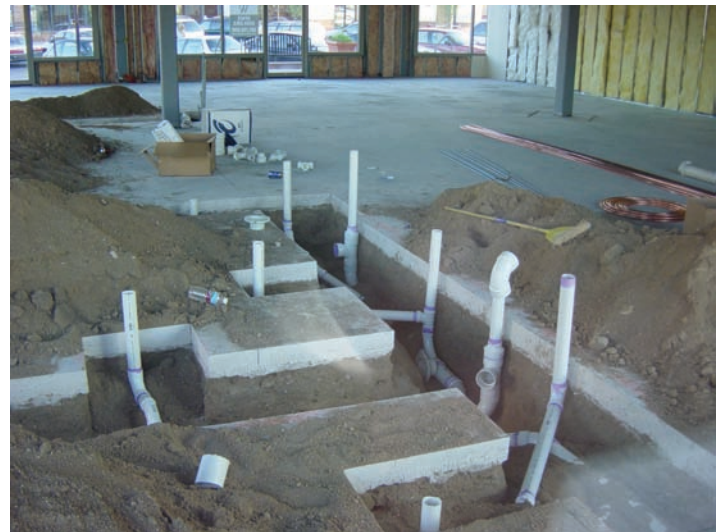
FIGURE 2-8 Underground plumbing must be inspected prior to replacing concrete
