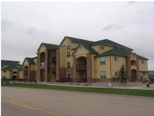
FIGURE 9-5 NFPA 13R sprinkler systems are limited to residential occupancies with a maximum of four stories
