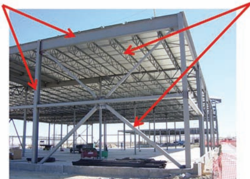
FIGURE 8-4 Primary and secondary structural members
