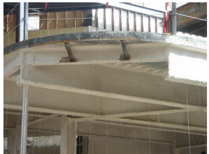
FIGURE 8-5 Sprayed applied fireproofing on structural members
