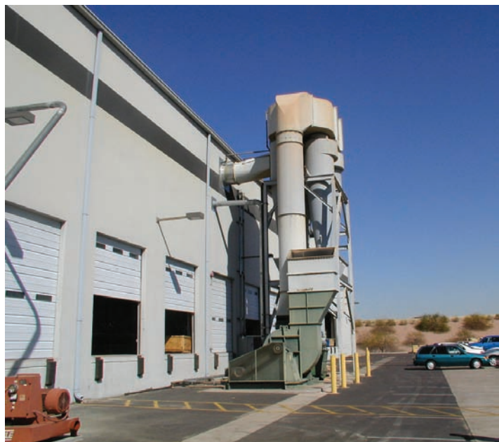
FIGURE 15-2 Dust collector used to capture combustible dust produced during the manufacturing of furniture
