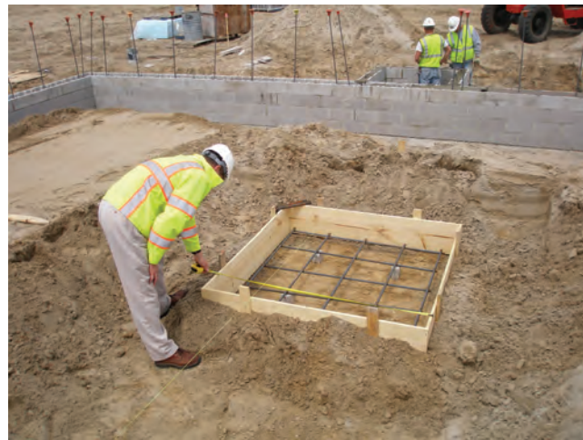
FIGURE 4-9 Inspection of footing
