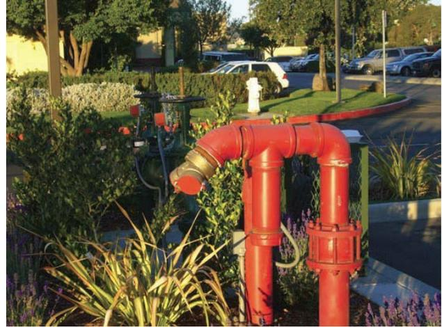
**FIGURE 9-13** Fire department connection for a wet-pipe automatic sprinkler system
