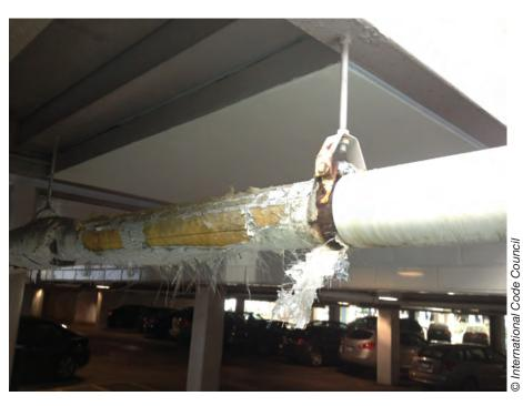
Even though this exterior piping insulation has been shielded from direct exposure to the elements by the structure above, it has still deteriorated.
