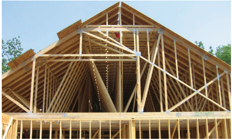
Uninhabitable attic with limited storage.
