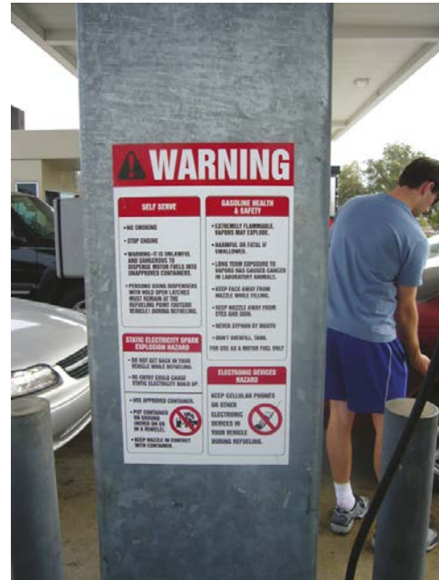
FIGURE 13-3 Dispenser operating instructions and warning statements are required for attended and unattended motor-fuel dispensing.
