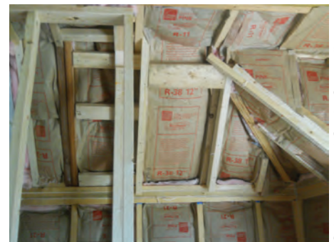
Insulation installed over eave baffles
