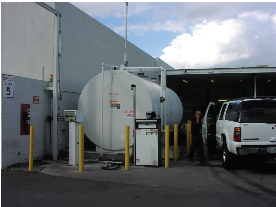
Flame arrester or PV breather valve required on protected above-ground tanks storing Class I flammable liquids
