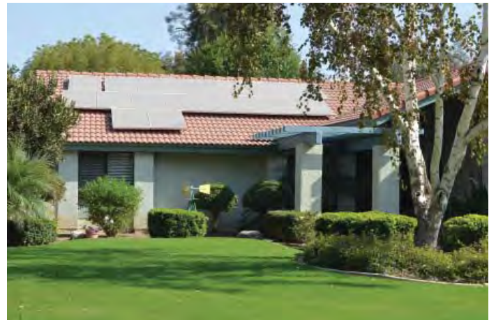
FIGURE 6-15 Solar panels on a one-family dwelling
