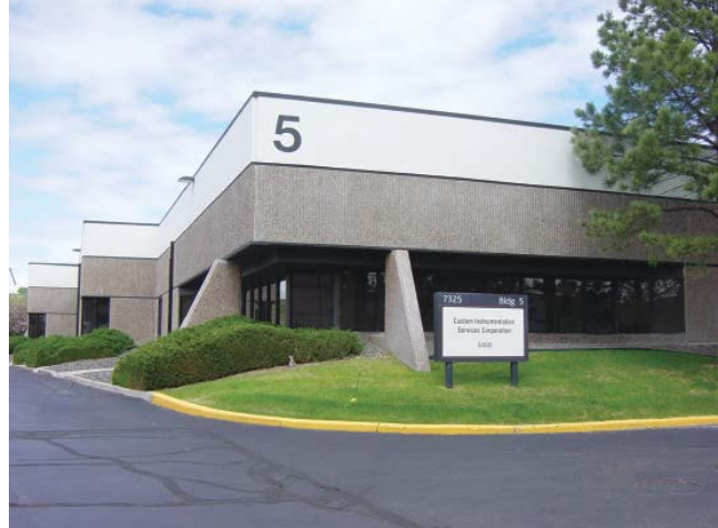
FIGURE 1-9 Existing building regulated by the IEBC
