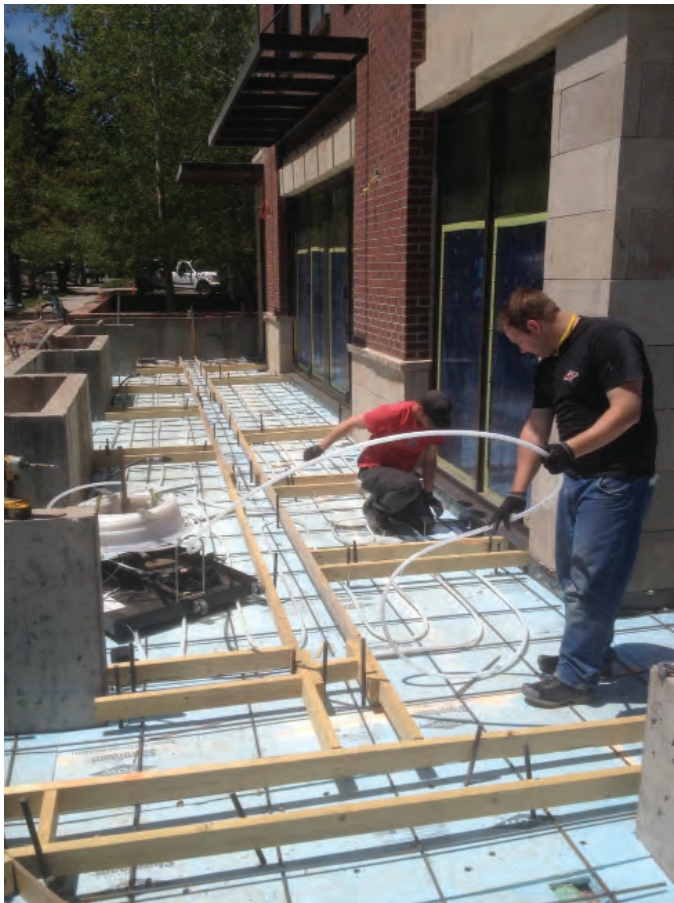
FIGURE 8-2 Snow and ice melt systems
