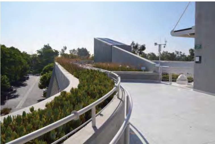
FIGURE 3-11 Landscaping on the roof must be maintained in a safe condition and allow fire-fighting access.
