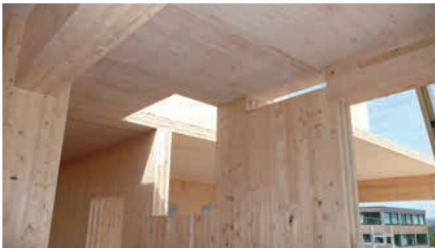
Cross-laminated timber construction.
