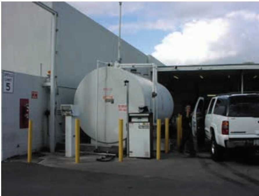
Flame arrester or PV breather valve required on protected above-ground tanks storing Class I flammable liquids
