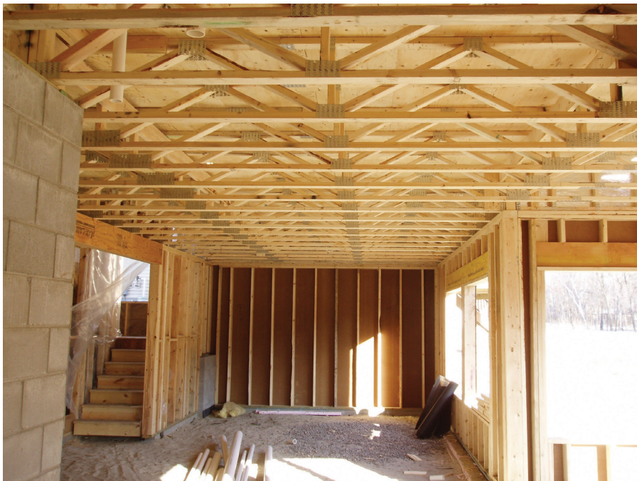
Open web floor trusses requiring membrane protection on the underside
