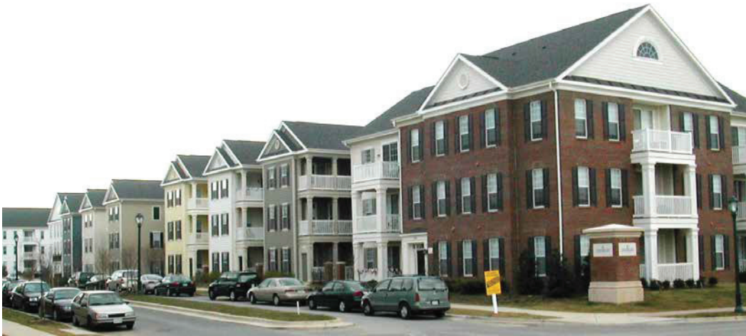
The Fire Service Membership Council succeeded in getting the ICC Board of Directors to support improved carbon monoxide detection and awareness in residential properties.
