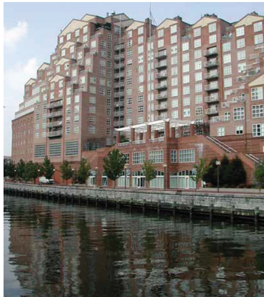
Limited access complicates firefighting and rescue operations. Circumstances like these are discussed at the Fire Service Membership Council to explore solutions and alternatives.
