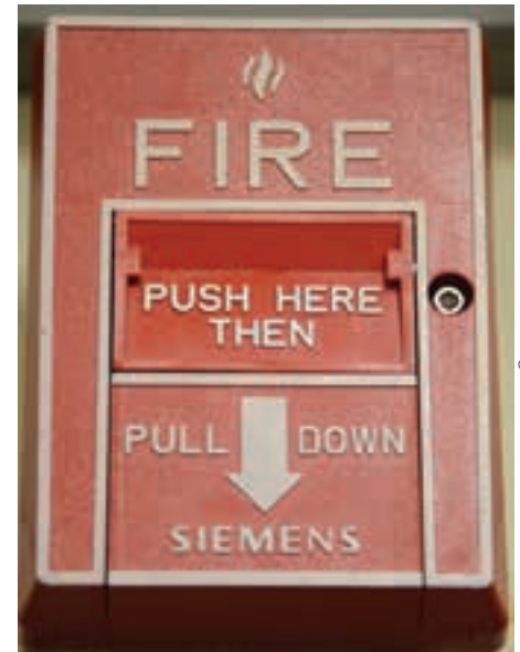
Manual fire alarm—double-action pull station
