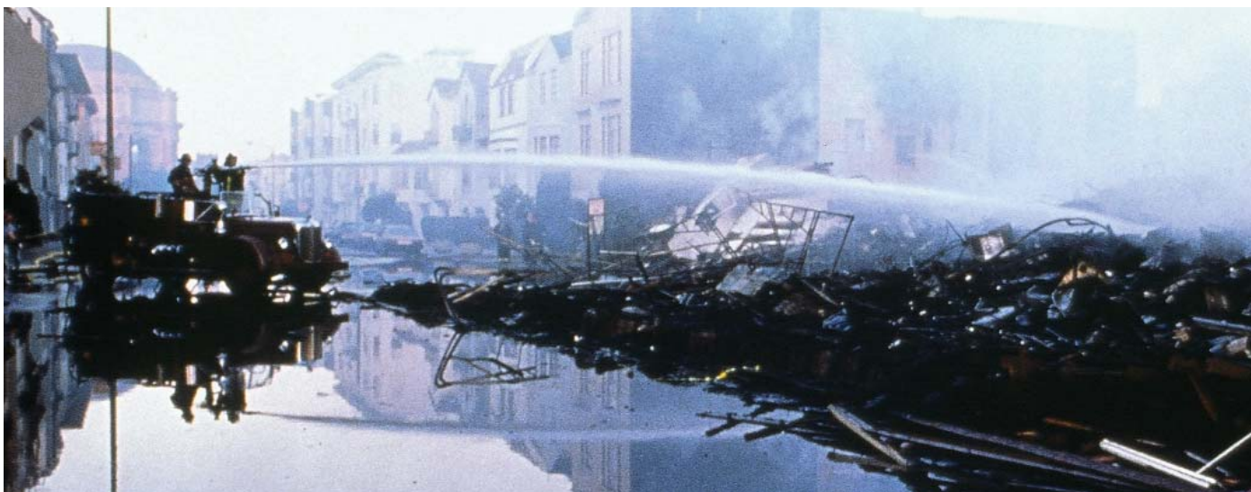
After the domestic and two separate underground fire service water systems experienced loss of pressure due to pipe damage, water had to be drafted from the San Francisco Bay by a fireboat to bring the 1989 Marina fire under control. (Photo by Mark Kluver.)
